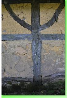
The cob is a mixture of water, clay and natural fibres (straw, hay, horse hair). It is used to fill half-timbered
